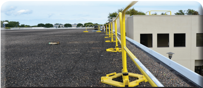
ROOF TOP SAFETY
